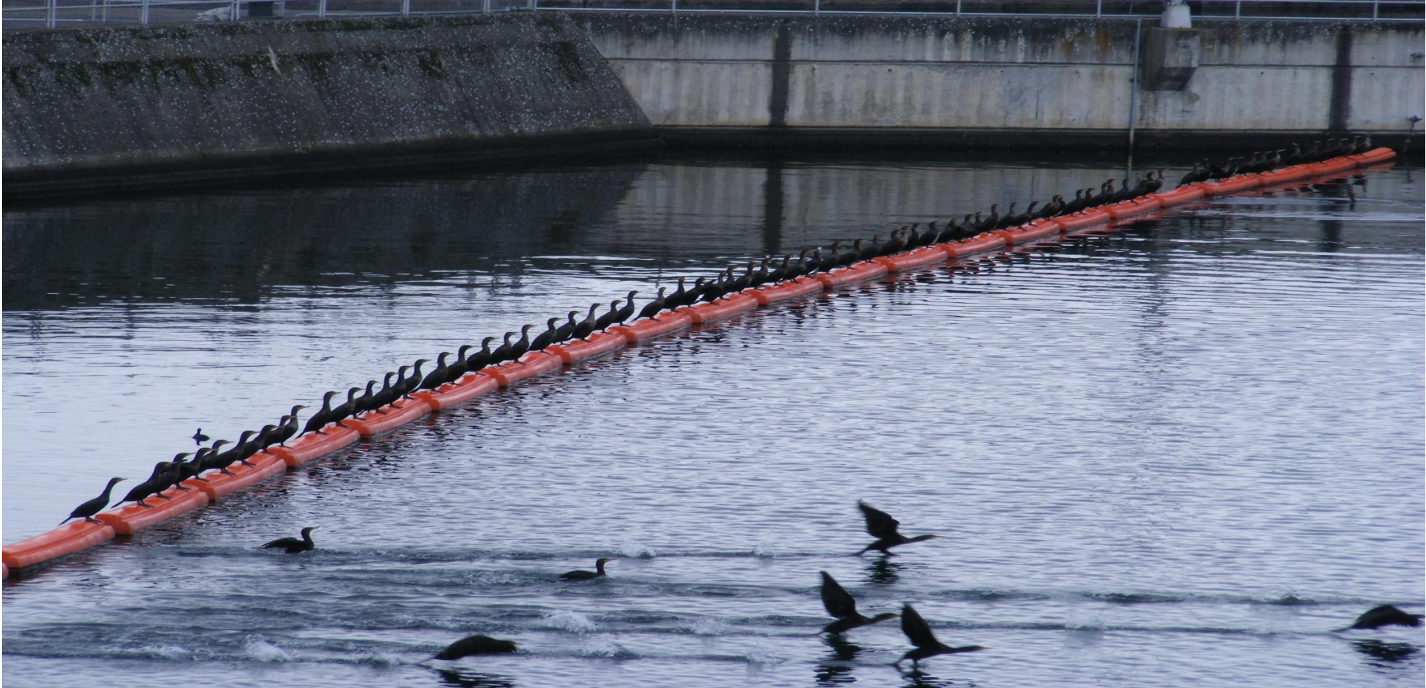
High Cormorant numbers resting on north forebay debris boom (~146)
